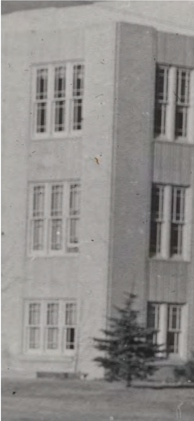
Glacier County Courthouse, circa 1945. North and east elevations detail, view to the southwest. Courtesy Glacier County Historical Society.
