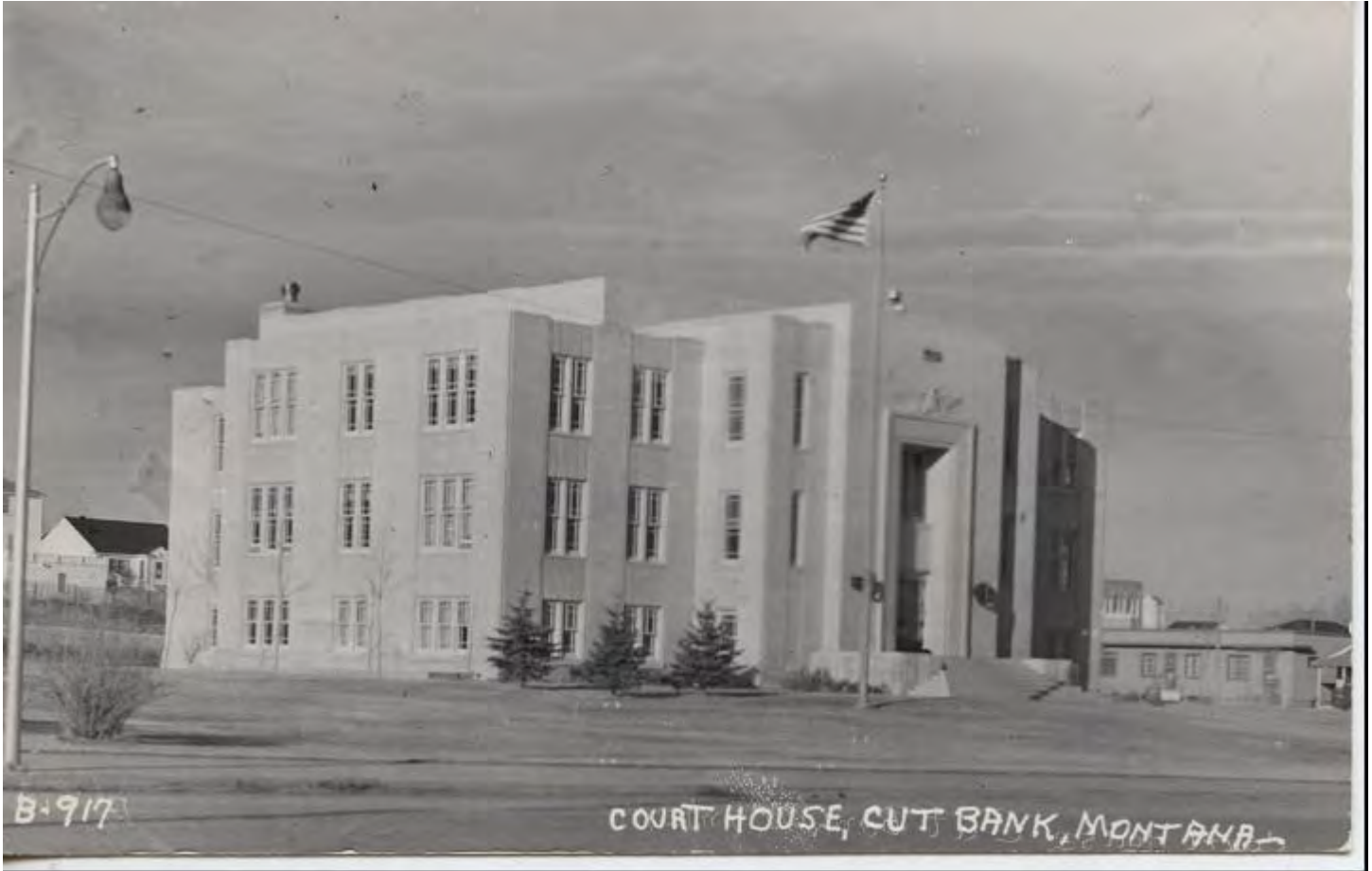
Glacier County Courthouse, circa 1945. North and east elevations, view to the southwest. Courtesy Glacier County Historical Society.
